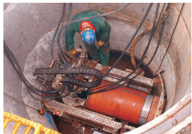
Auger Boring in the UK
